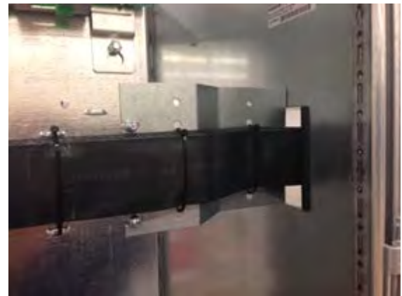
Figure 5-14. – Typical Ribbon Cable Routing Between Enclosures
