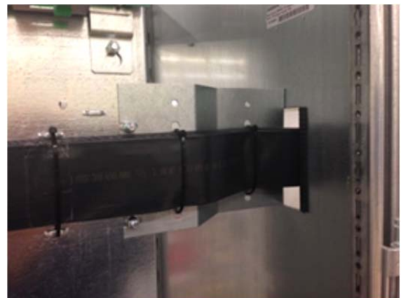
Figure 5-19. – Typical Ribbon Cable Routing Between Enclosures
