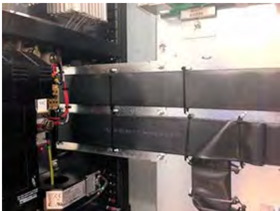
Figure 5–18. – Typical Ribbon Cable Routing Across The DELTA Transistor Modules
