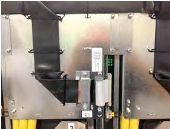
Figure 5–16. – Ribbon Cable Clamp At The DELTA Transistor Module
