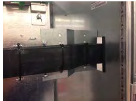
Figure 5–19. – Typical Ribbon Cable Routing Between Enclosures
