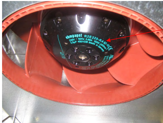
Figure 4 Fan part number on motor
